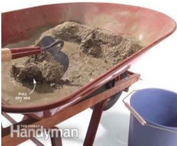
Photo 3: Gradually wet the mix
