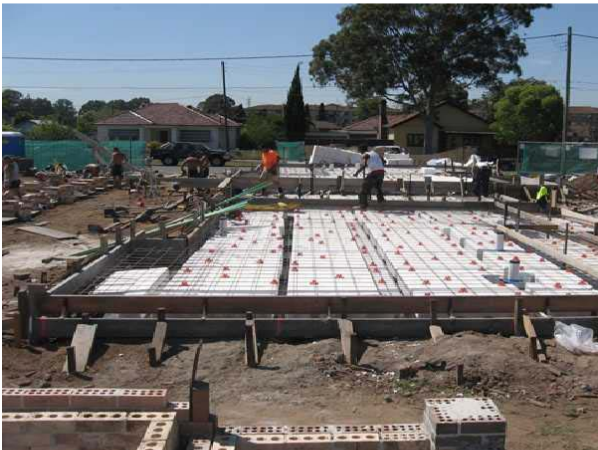
Waffle slab example
