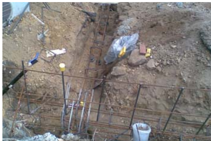
Trenches with reinforcement for strip footing
