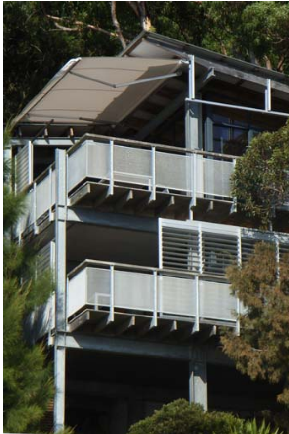
Steel pole house with exposed structure
